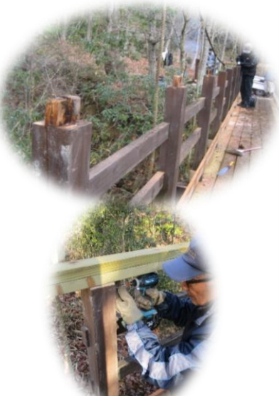
20 (R2) 07.04 床板・手摺の腐食が激しく散策に危険な木橋
